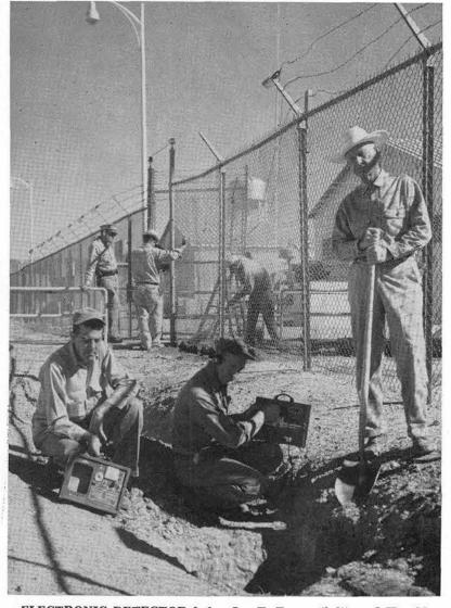
ELECTRONIC DETECTOR helps Joe T. Evans (left) and Harold Neuhaus (both 4514) locate underground pipe south of Personnel Bldg. Lee Brazell (4575) stands ready to dig at exact spot.
